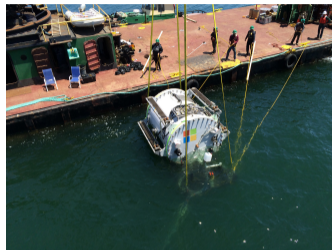
Microsoft's project Natick: immersed datacenter
